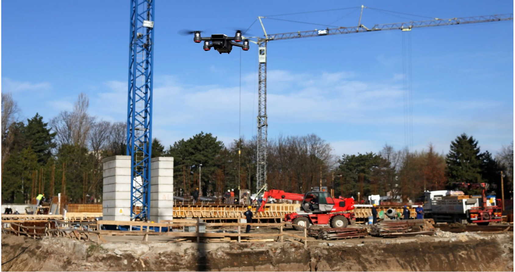
Monitoring the progress of construction project
